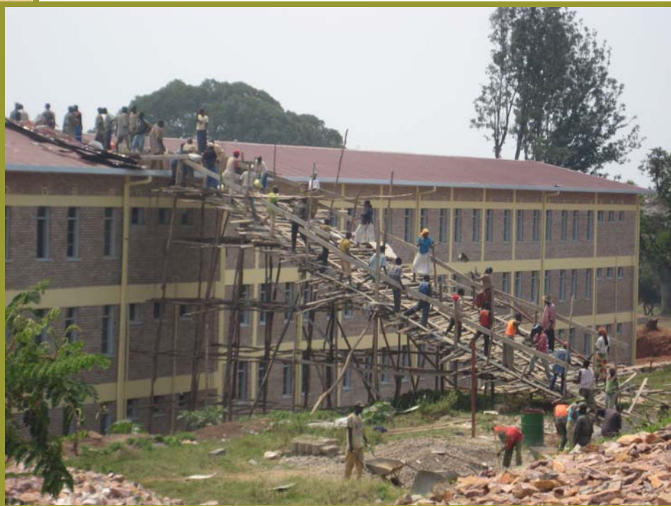
Building a dormitory at the National University of Rwanda, Butare, Rwanda
